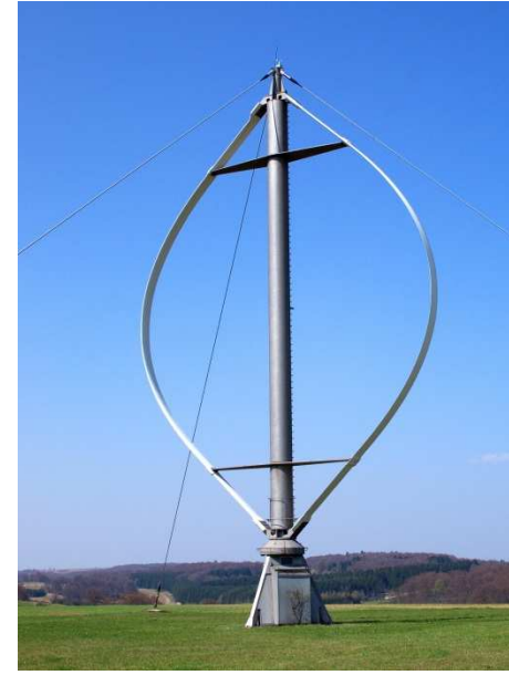
Darrieusova turbina
